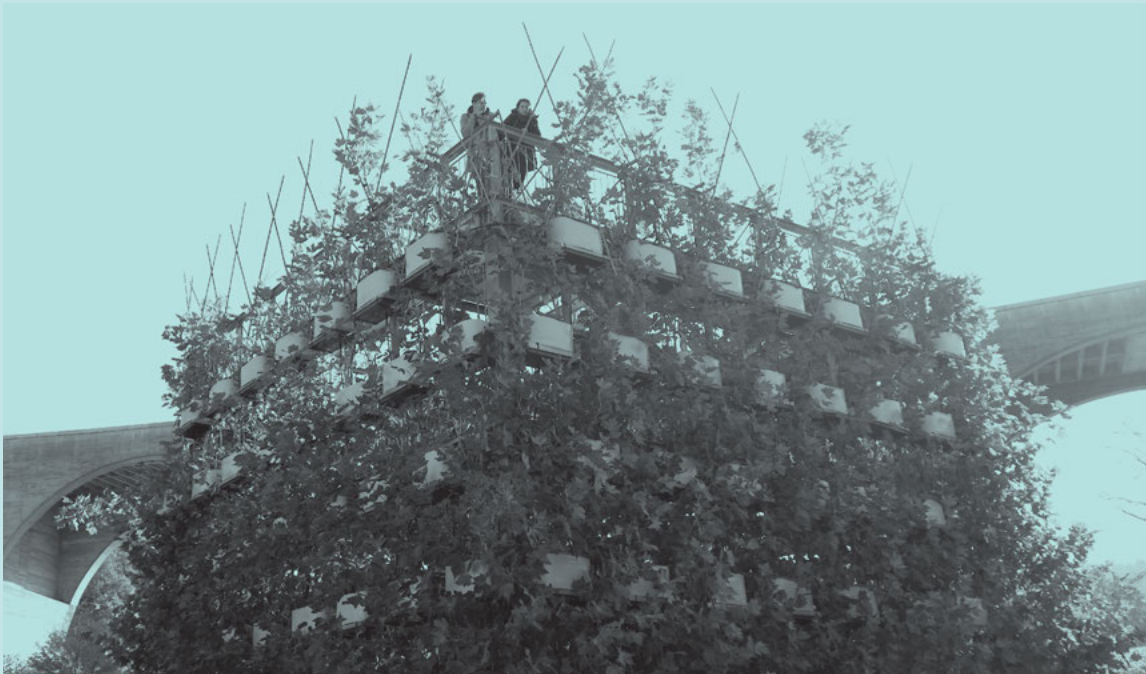
▲ ▲ Fig. 5 | Abb. 5: Left: Plane Tree Cube in Nagold, Germany by OLA – Office for Living Architecture. Right: Joint trees that will develop into the main load-bearing structure. Photos © Ferdinand Ludwig
